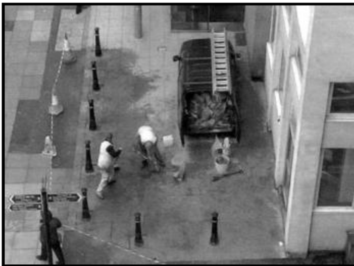
Contractors Parking Problem
